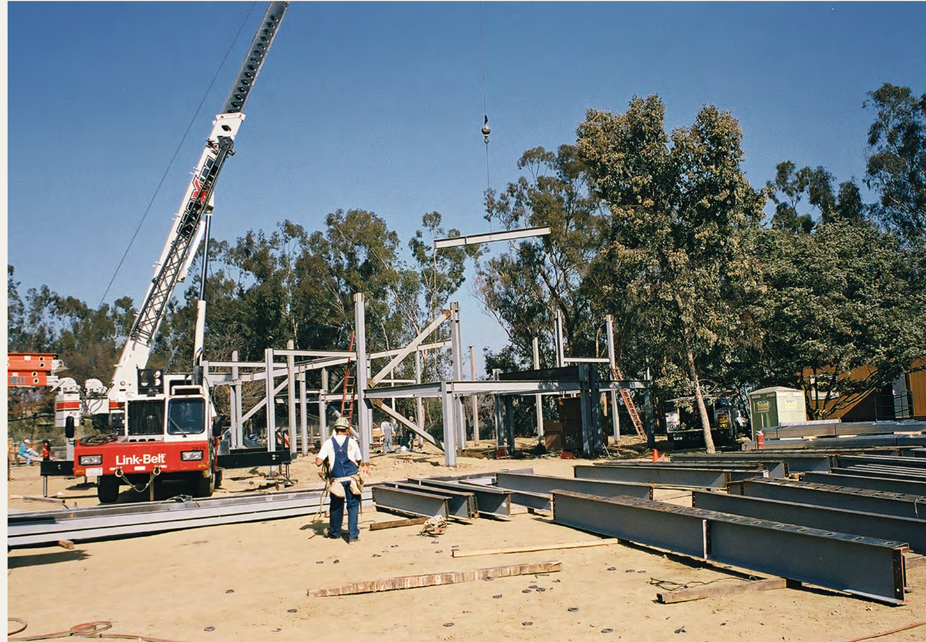
Construction of the Schuman Family Foundation Conference Center and underground cistern (2004)
