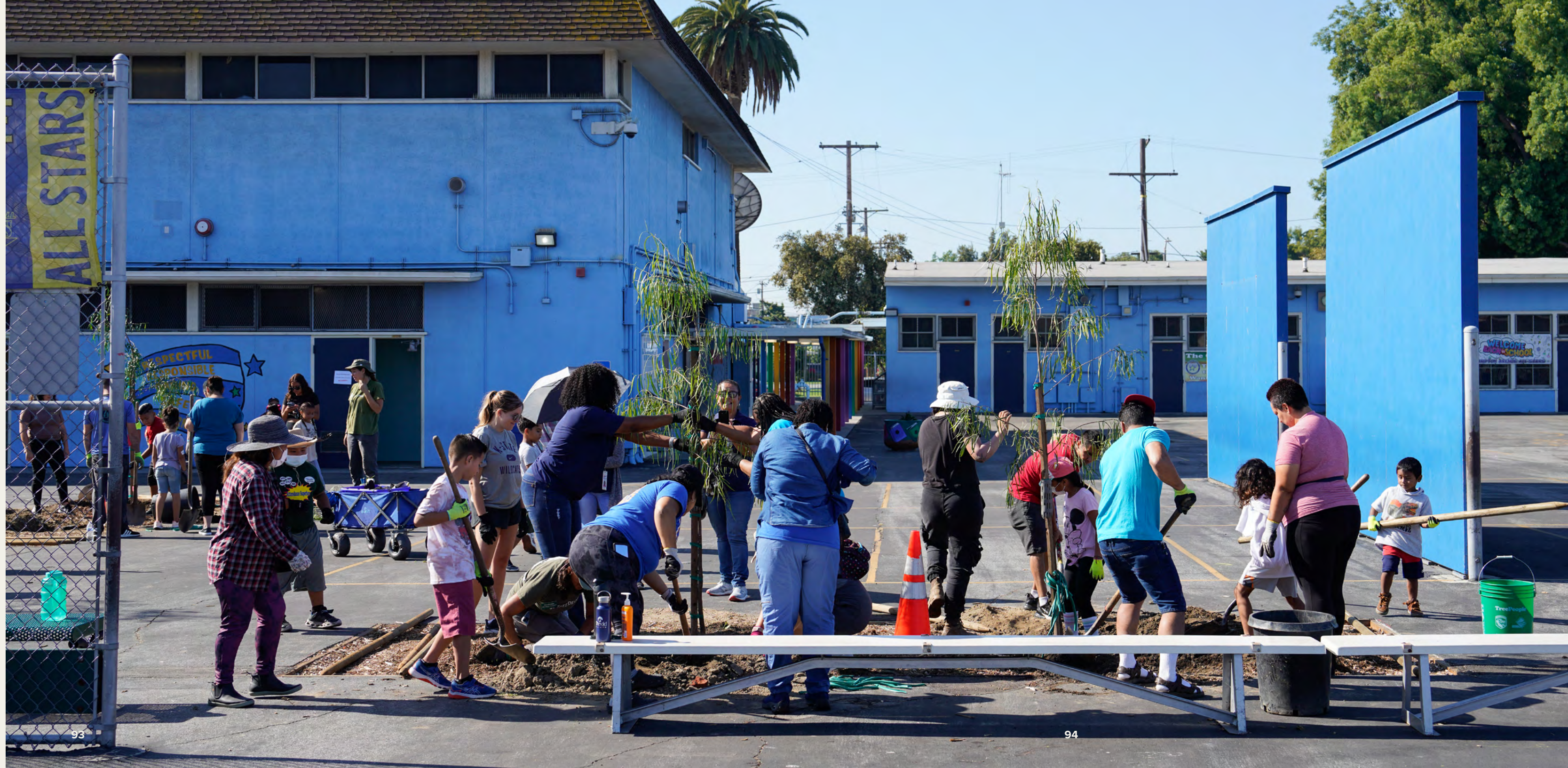
At Compton Elementary School, TreePeople removed asphalt to create space for shade trees and planted 21 trees with 65 volunteers. (2023)
