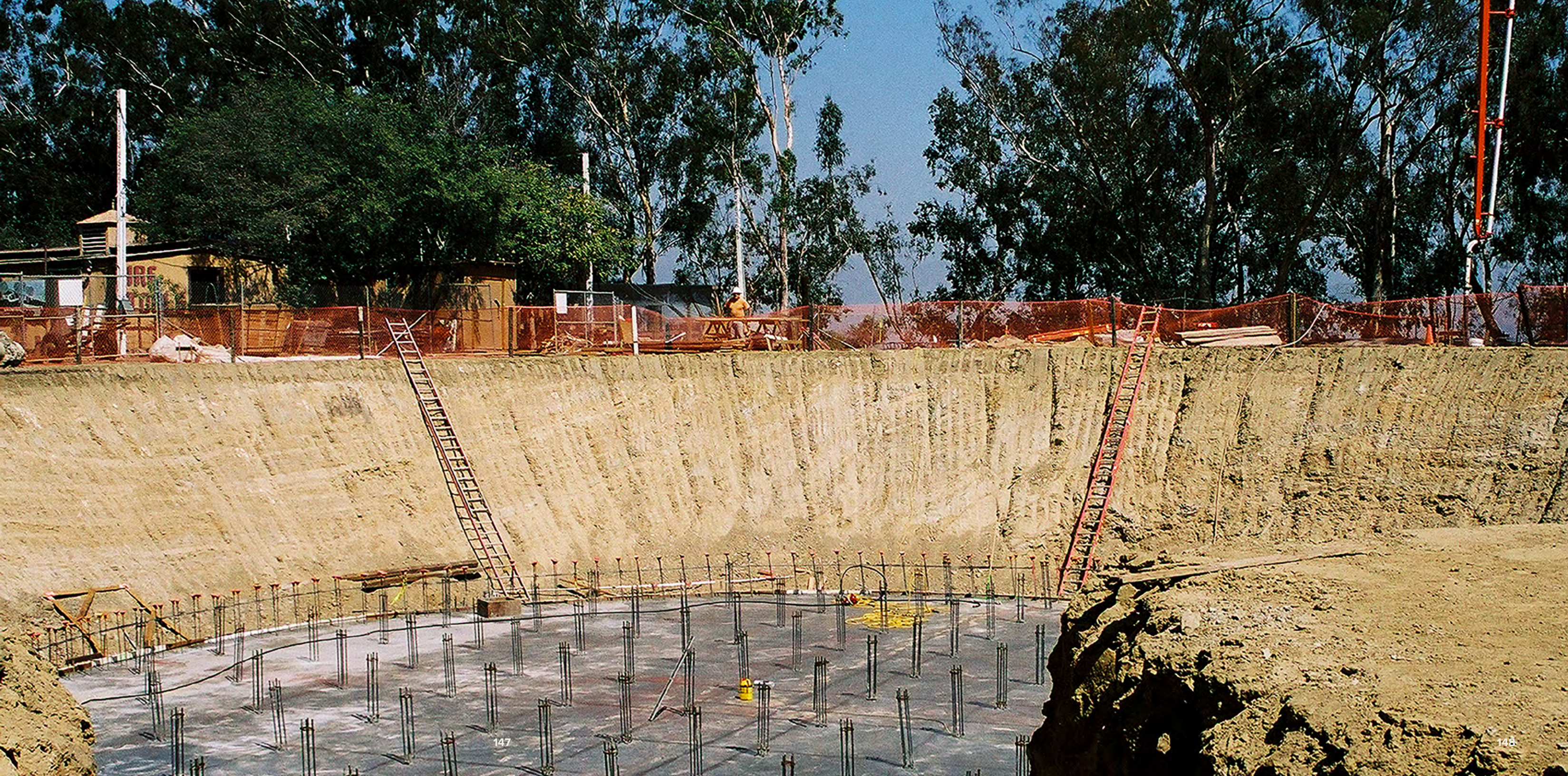
Construction of the underground cistern that stores rainwater for the site. (2004)
