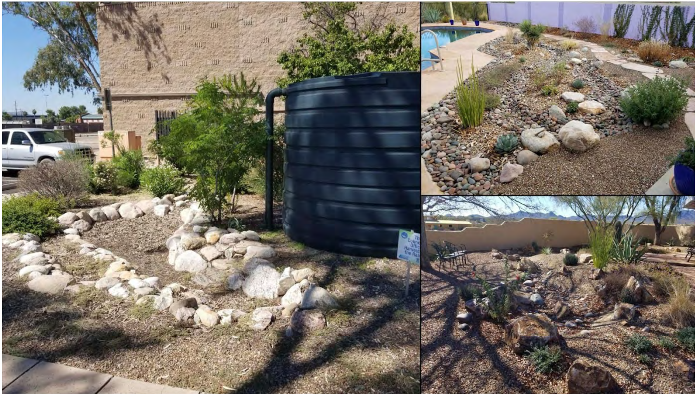
Figure 18: Images of Passive System Galleries in Tucson. The photo on the left displays a system reinforced with rocks and a direct overflow feed, the top right photo displays a system with a direct downspout to feed bioswales, and the bottom right photo displays a system with minimal rocks and a direct feed. Pictures from the City of Tucson .
