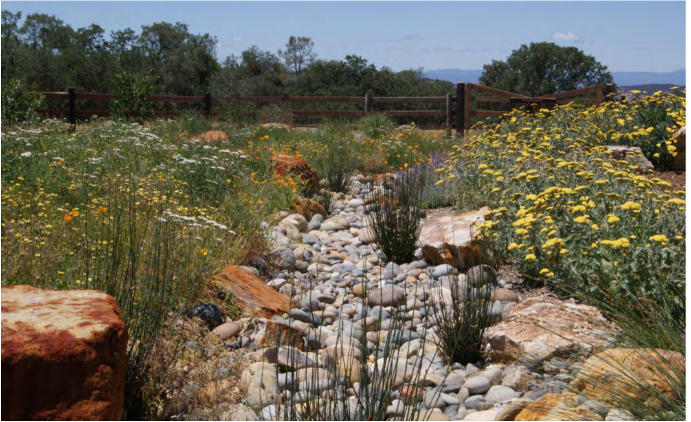
Figure 14: Swale with similar visual appearance to a Native Dryland Bioswale demonstrating use of California Native Plants (Credit: Madrone Landscapes)
