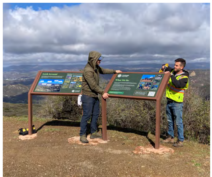
New Lois Ewen Overlook interpretive signage installation
