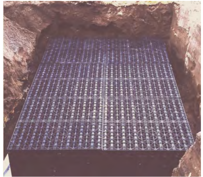
Left: Stormceptor oil/sediment filtering device installation
