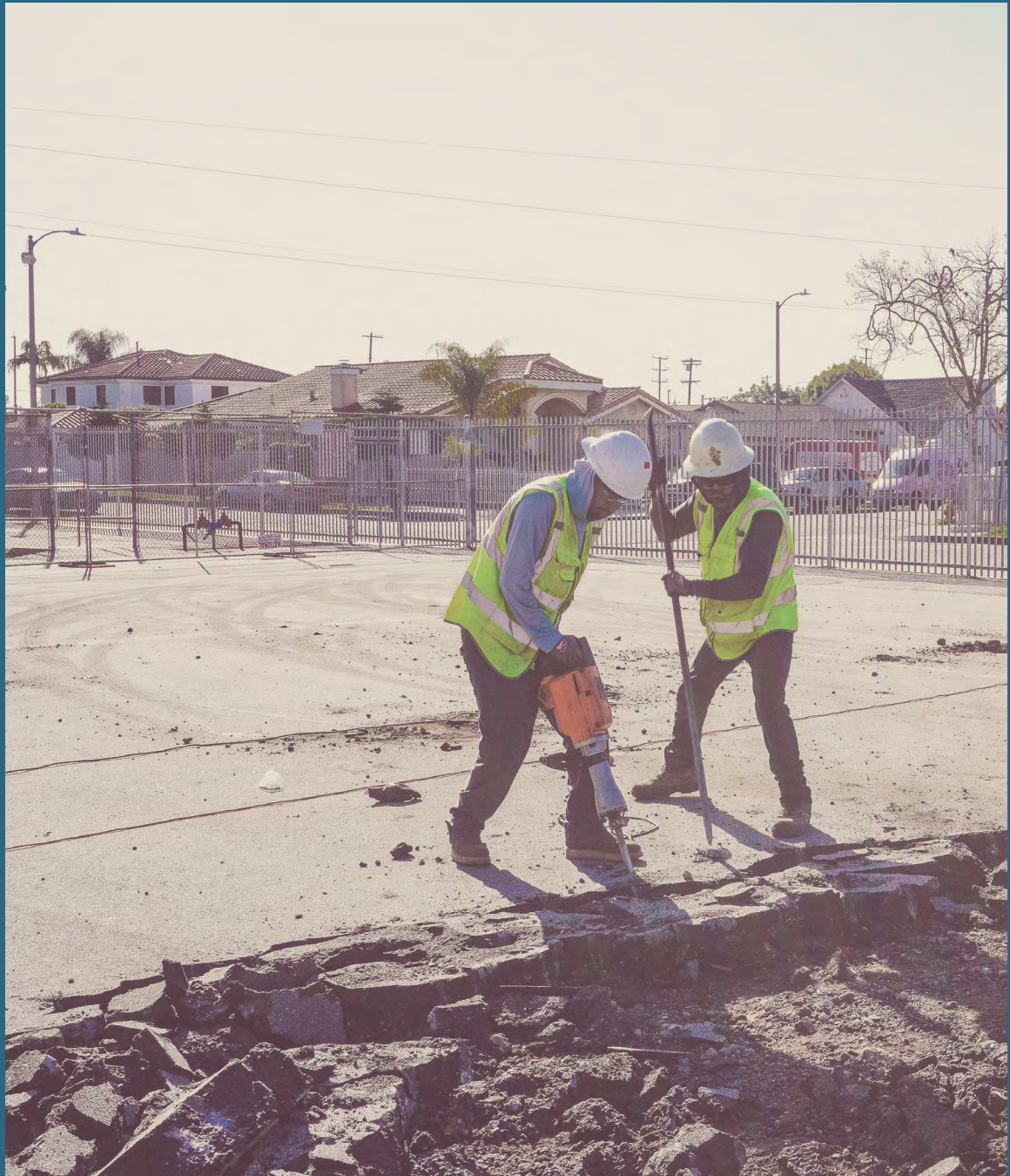
Wilmington Middle School asphalt removal Photo credit: Kai McDaniel
