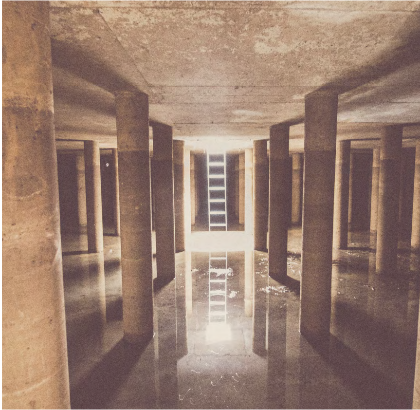
Coldwater Canyon Park Cistern
