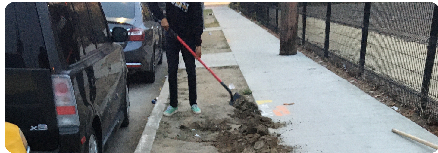
Figure 1 - A study team member begins preparing a tree well within a 3.5 feet diameter parkway
