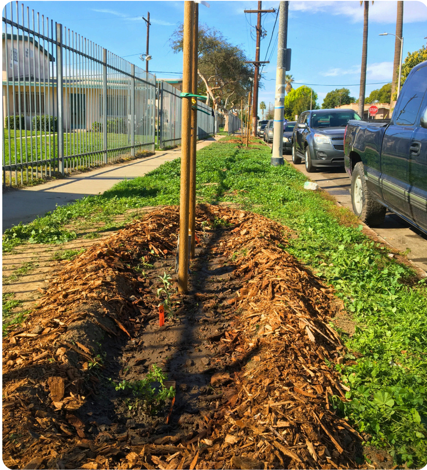
Figure 11 - A tree planted with California native companion plants within a shared berm and a layer of mulch ground cover. All native ground cover were transplanted from 4" nursery pots. The turf growth seen in this image was not present until after the installation and watering of trees and soil treatments.
