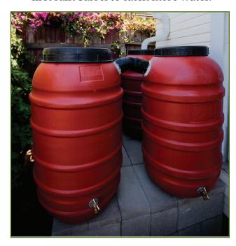
3. If the downspout runs along a wall, it will need to be shortened and have an elbow attachment added to extend out to the top of the rain barrel.
